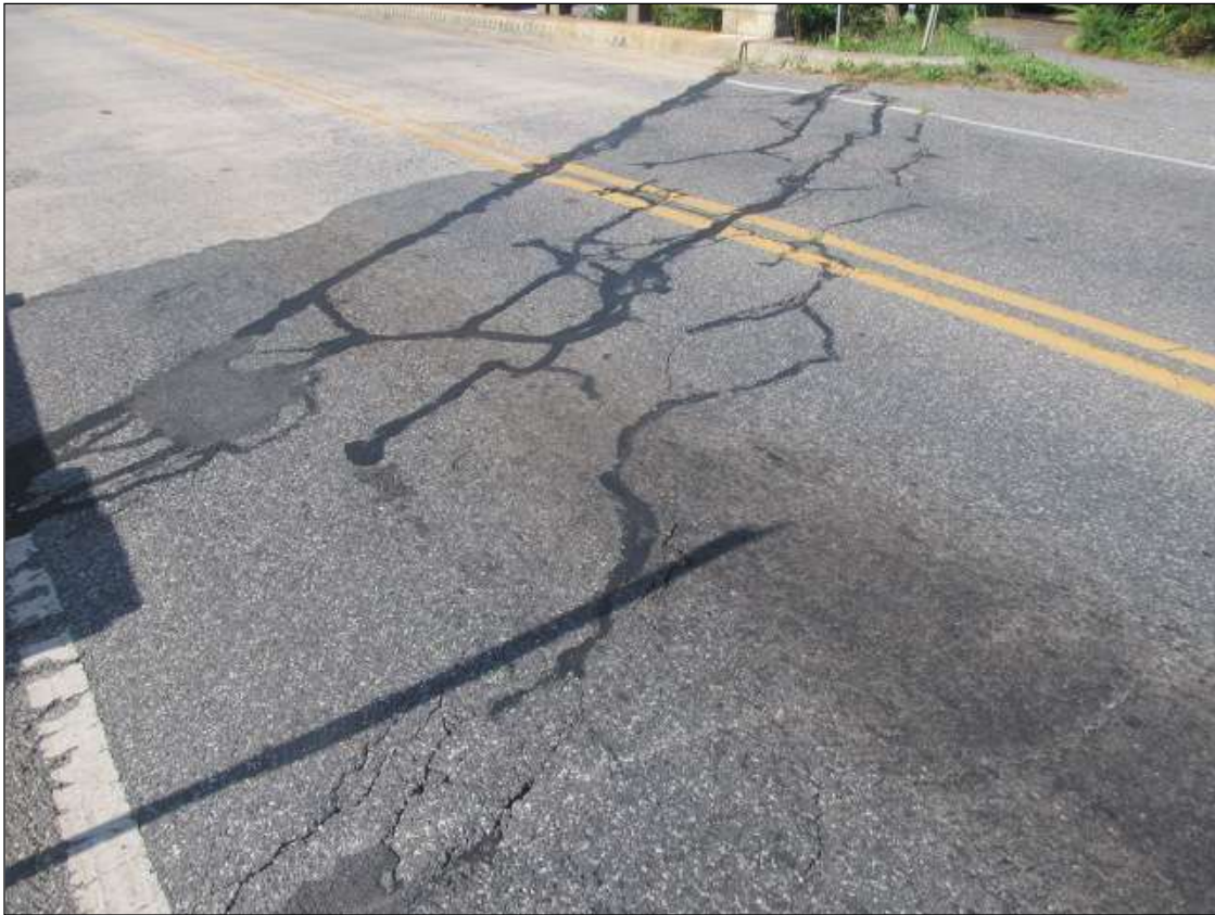
THE APPROACHES ARE SETTLED 25' WIDE X 8' LONG X 1" DEEP ALONG THE FILLFACE.
