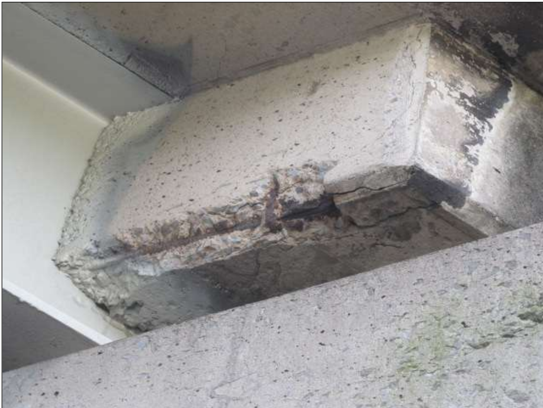
THE EXTERIOR DIAPHS. ARE CHIPPING ALONG THE BOTTOM CORNERS WITH REBAR EXPOSED.
