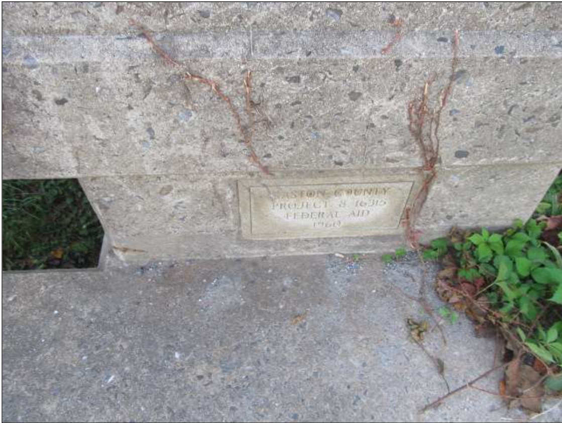
BRIDGE INFOR. MARKER AT THE SOUTHWEST CORNER
