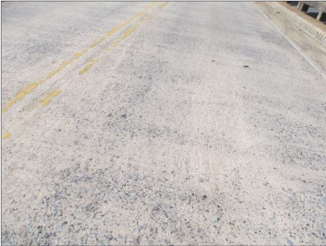
TRANS. CRACKING PRESENT IN SPAN 4
