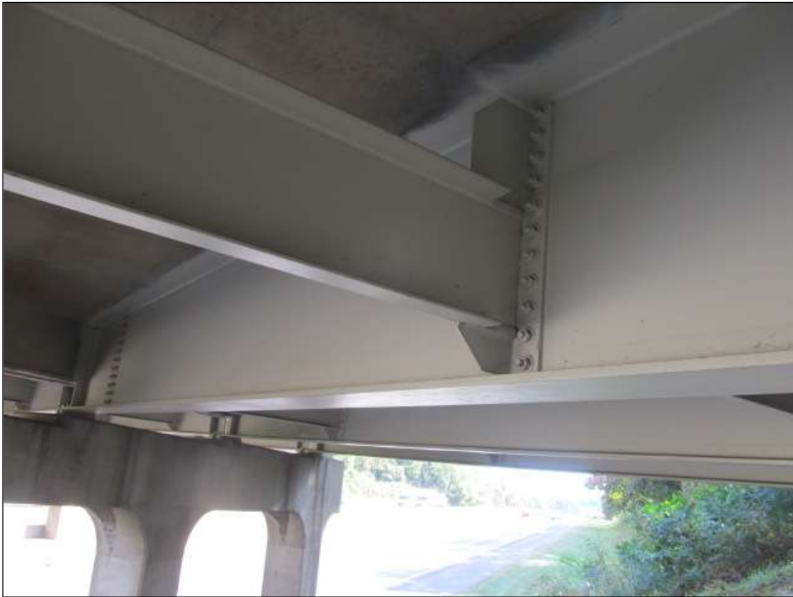
BEAM. AND DIAPHS. PAINTED CODED I.
